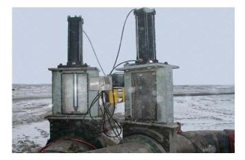
Special hydraulic cylinder sensors designed to operate in temperatures as low as -50°C (-58°F) are available. These products feature polymer materials designed and specified to operate down to those temperatures. To combat electronic malfunction under these conditions, the manufacturer may specify that power should remain applied to the electronics at temperatures below -40°C (-40°F). The heat dissipation of the electronics themselves keeps them within normal operating limits.
